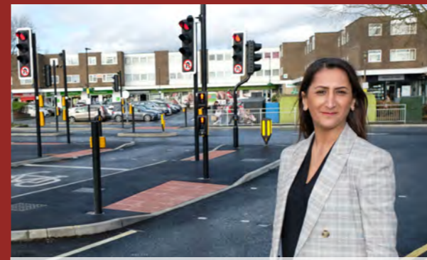
Bally Gill (Langley St Mary's) at the junction widening and road improvement works on Langley High Street - a major highway infrastructure scheme delivered by Slough's Labour-run Council.
