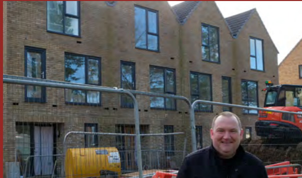
Martin Carter (Britwell & Northborough) views 12 new Council Homes constructed on Wentworth Avenue - 575 social & affordable homes will be built in the next round of Slough Council's capital programme.
